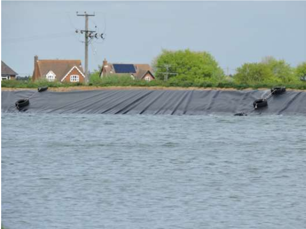
Reservoir, Hams Farm
