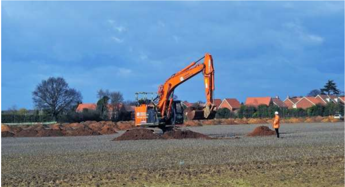
Digging Trenches ( not a trowel insight)
