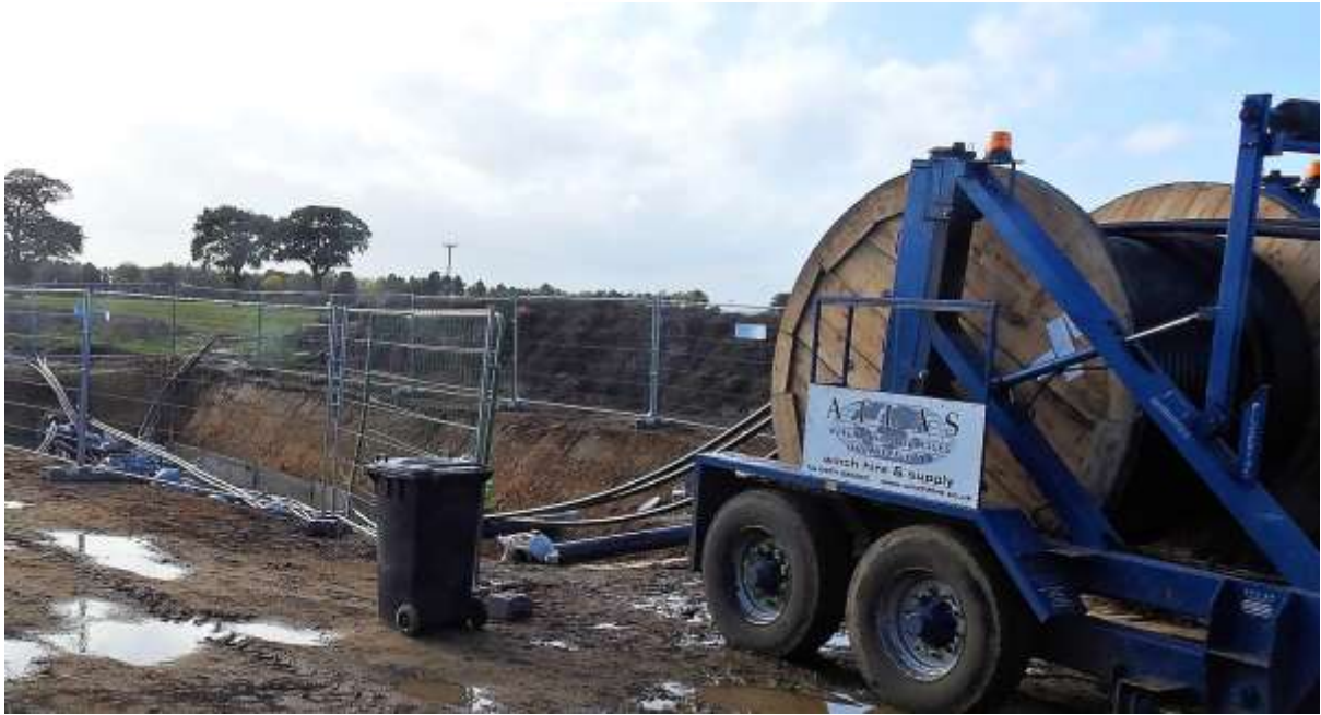
Laying Power Cables, Grimston Lane
