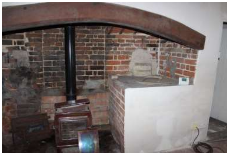
The kitchen hearth with the built-in copper on the right and a patchwork of bricks behind.
