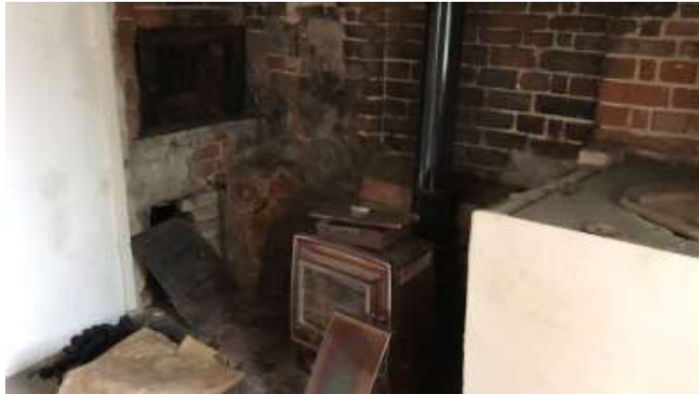
The Bread oven built in to the other side of the kitchen hearth.
